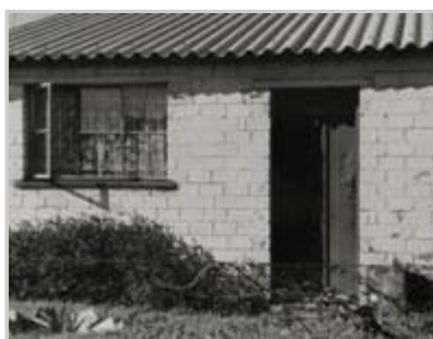
House, 901A Zola.
