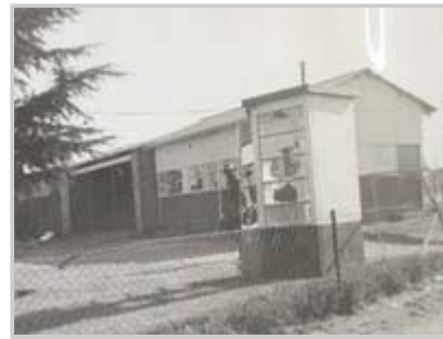
Damaged building and telephone booth, Orlando West.
