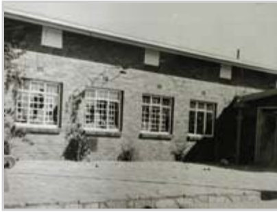
WRAB office outside, Katlehong.
